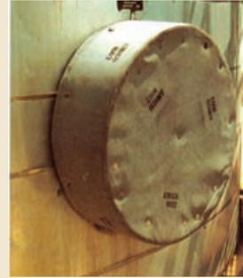
*Semi-rigid RE/WRAP insulation cover, installed over man way on heated storage tank, guards against inadvertent worker contact with elevated temperatures*
