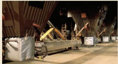
*RE/WRAP insulation covers enclose ash-handling equipment and controls beneath 144 precipitator hoppers at this coal-fired power plant, guarding operating personnel against contact with elevated temperatures. Insulation covers are of silicone-impregnated fibrous glass fabric for wear resistance*
